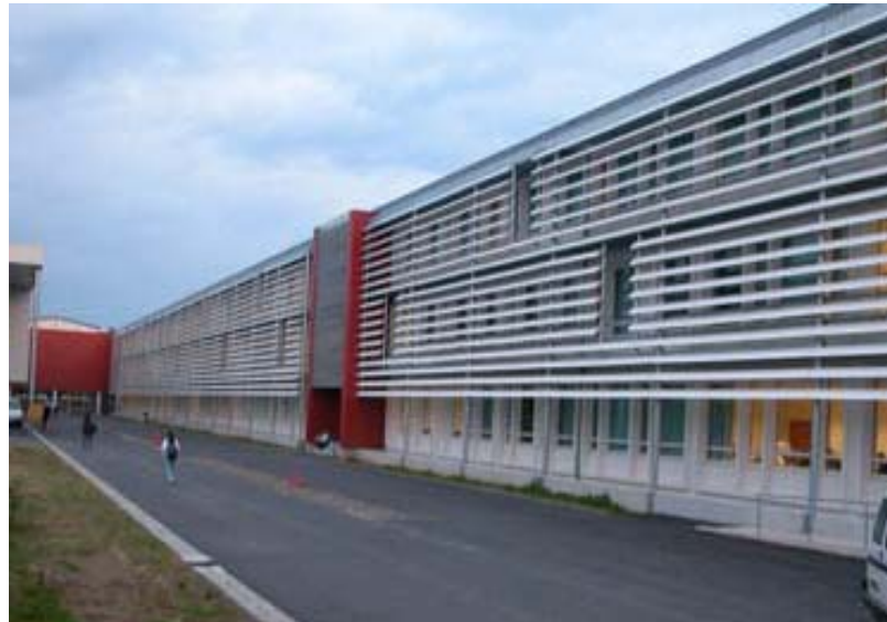
Figure 3.2: Strategies to improve energy efficiency in non-domestic buildings. Shading devices fitted to Lycée Chevrolier, a high school in France (above), and solar shading and natural lighting, Jubilee Campus (below)
