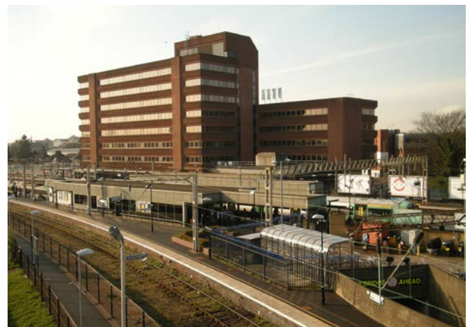
Fig 46 Watford Junction station
