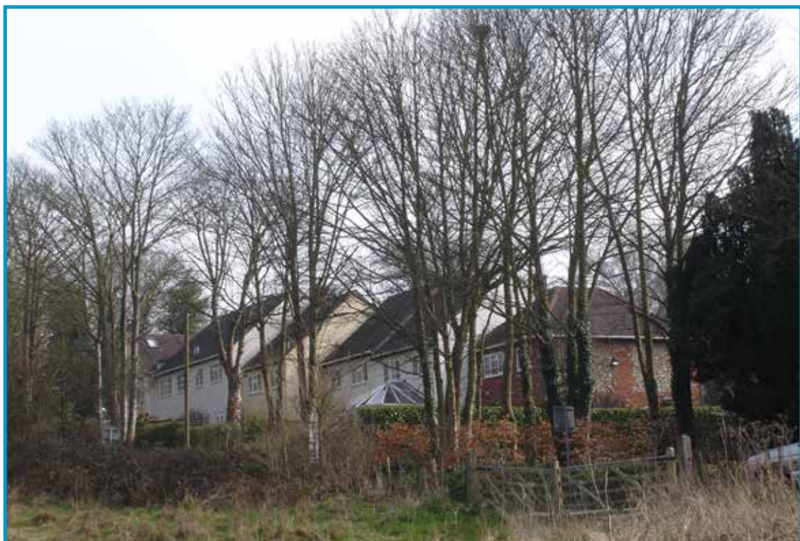
Nos.1-7 Heath Farm Court viewed from the north
