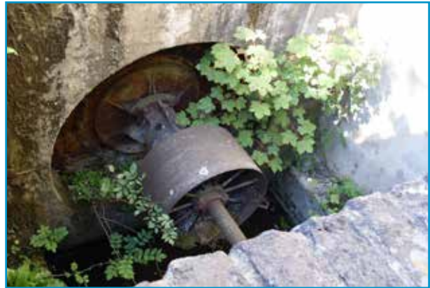
Turbine remains in a wheel house
