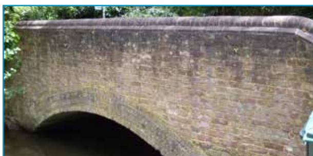
Road Bridge over River Gade
