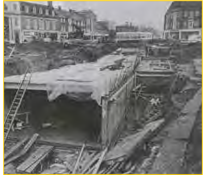
Underpass under construction
