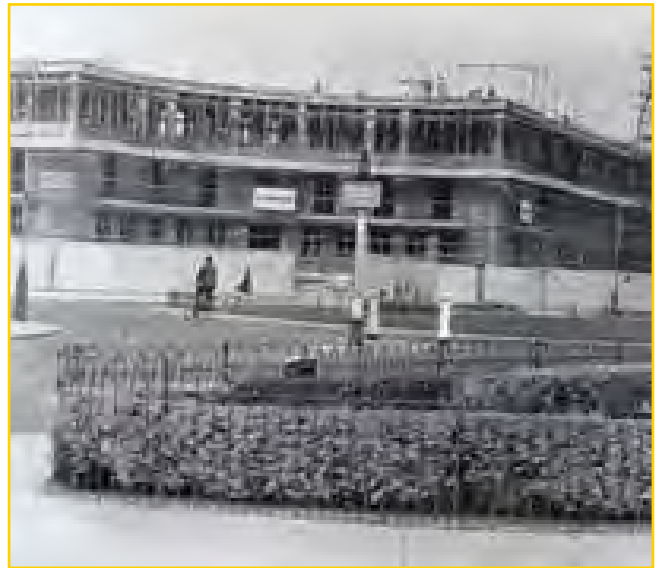
Town Hall under construction
