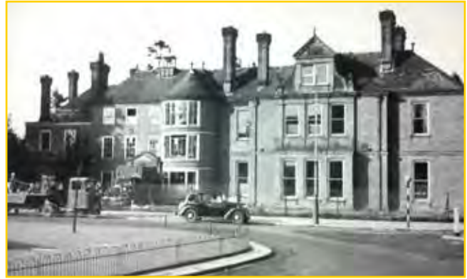
The Elms prior to demolition
