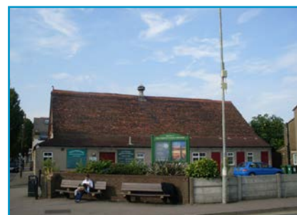
Note attractive roof and ridge tiles on this chapel
