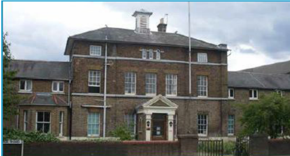
The former Watford Union Workhouse on Vicarage Road
