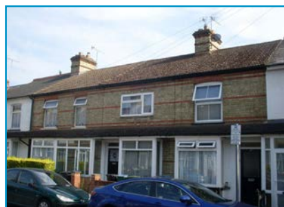
Inappropriate alteration of historic window opening
