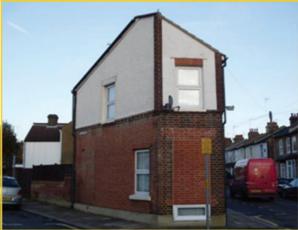
Poorly designed conversion
