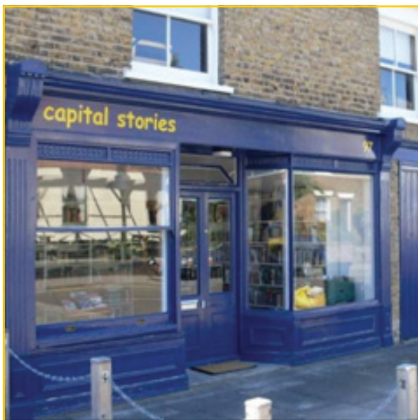
Traditional design of shopfront In Oxhey
