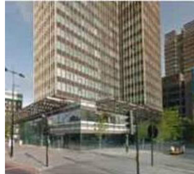
Use of terraces and awnings to prevent wind impacts
