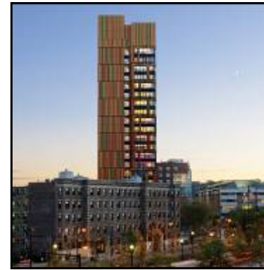
Good example of different materials and cladding on an existing tall building
