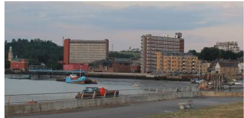
Slab Block Building with large bulk creating a significant visual impact (Mountbatten House and Anchorage Building, Chatham Kent)
