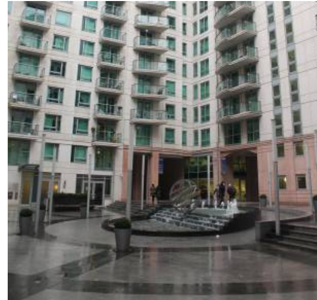
Disabled access needs to be integrated into the design – St. George's Wharf
