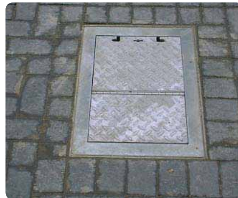
POWER BOX - IN-GROUND SUPPLY
