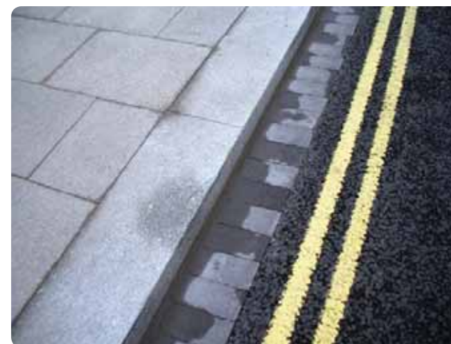
Carriageway kerb line
