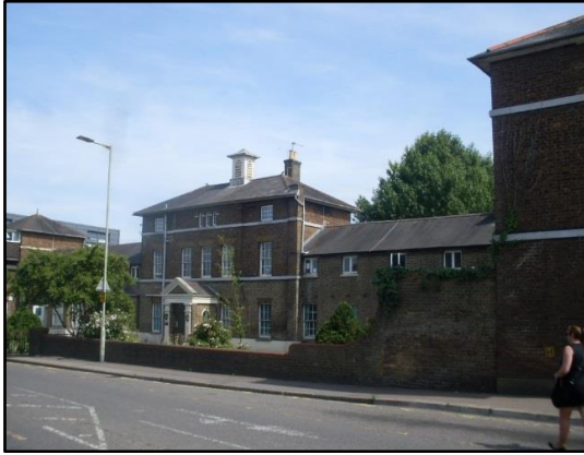
Administration Block at Watford General Hospital
