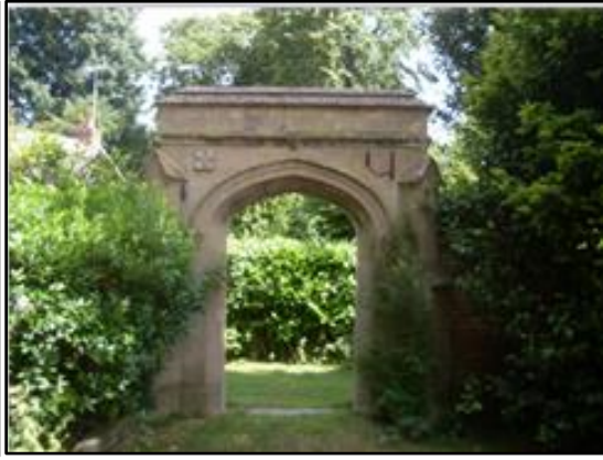
Gateway and attached lodge walls approx 30m northwest of 24 The Gardens
