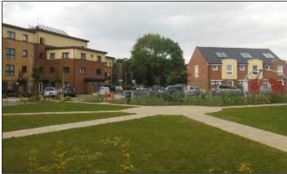
Figure 9-1: Former Fire & Ambulance Station development, Whippendell Road
