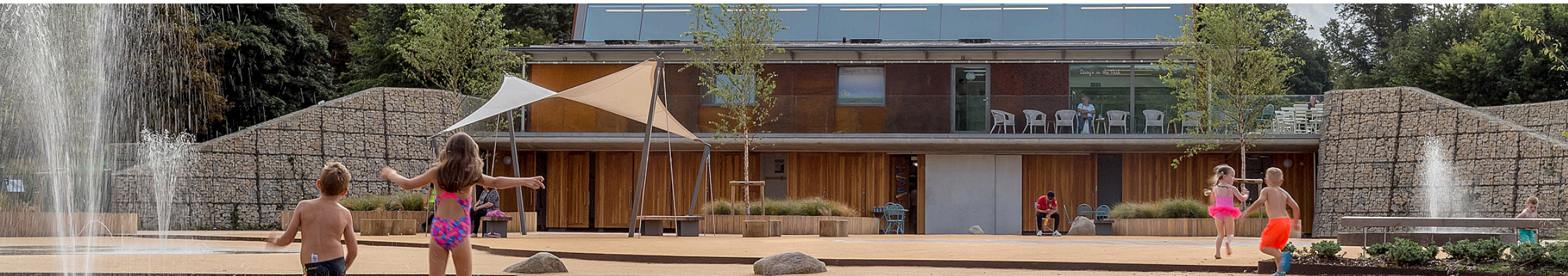
Cassiobury Park Hub © Knox Bhavan Architects for Watford Borough Council / Building Futures Award 2018
