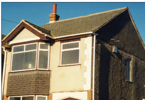
Closer view of main windows
