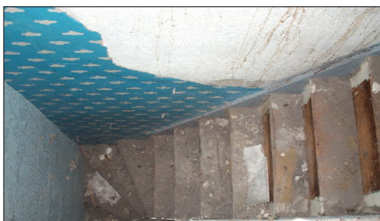
View of stairs from landing
