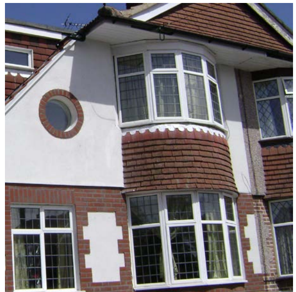
This is an example of an insulated Watford property that used a combination of smooth render with a brick finish.
