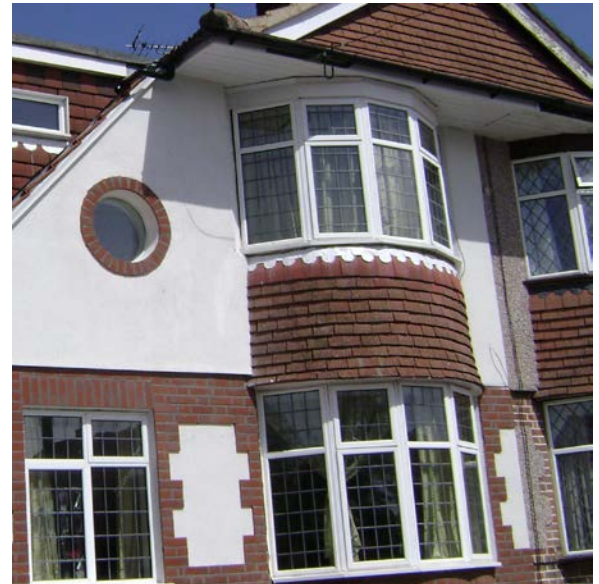
This is an example of an insulated Watford property that used a combination of smooth render with a brick finish.
